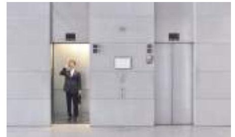
Elevators Preventive Maintenance
